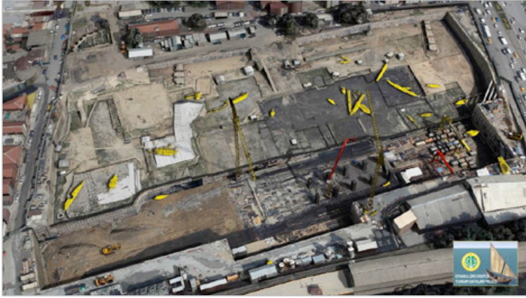
Fig. 1 View of excavations at Yenikapı, former Theodosian Harbor and shipwrecks.
